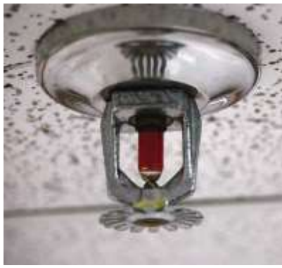
An example of a commercial fire sprinkler
